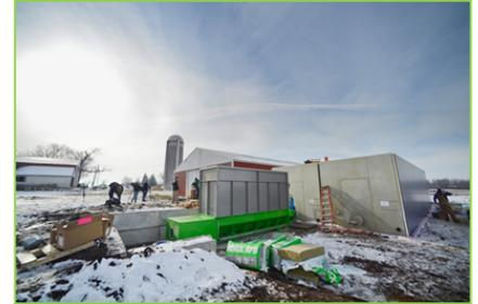
The Allen Farms digester project and technology, referred to as the “Titan64” or the “EUCOLino” (OY-co-lino) conducted by BIOFerm™ Energy Systems and the University of Wisconsin Oshkosh, involves the first small-scale biodigester unit in Wisconsin. It is an innovative, scaled technology involving wet digestion and a 64kW engine using plug flow system technology.
